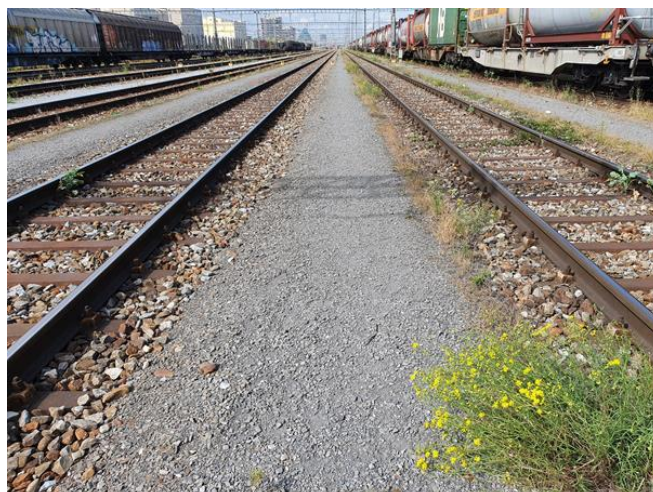
Figure 5: SBB - Track on the left: Treated with hot water. Track on the right: Not treated. The species type is Senecio inaequidens . Taken by Lukas Tanner on September 22 nd , 2020
