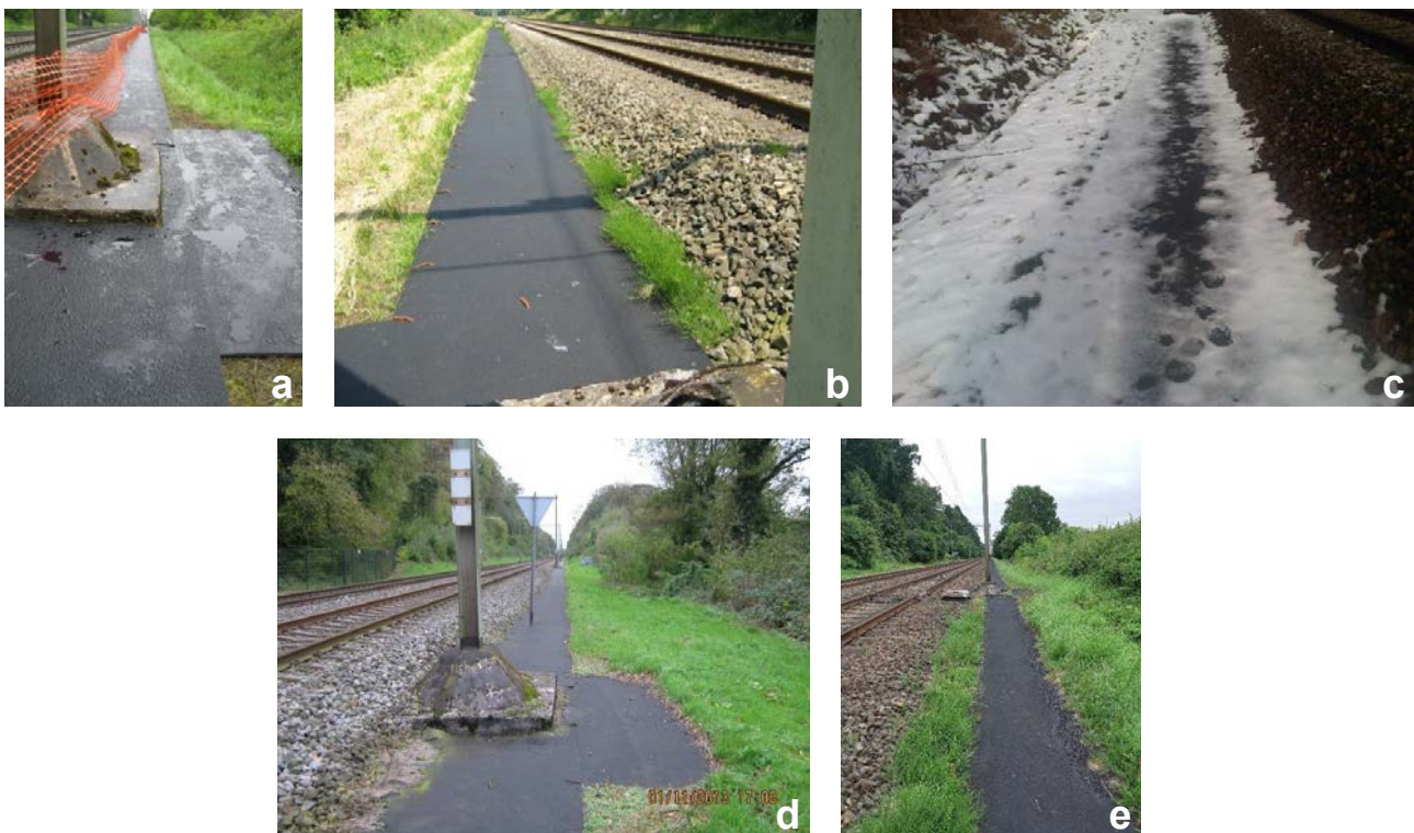
Figure 12: Anti-vegetation mats - ProRail (a) October 2009, (b) June 2010, (c) December 2010, (d) November 2013, (e) July 2019
