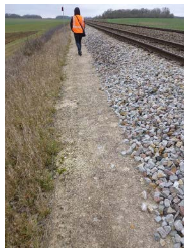
Figure 51: Geotextile laying and covering after 5 years
