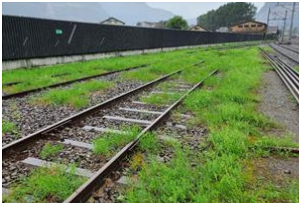
Figure 24: SBB Hot water case study - before treatment
