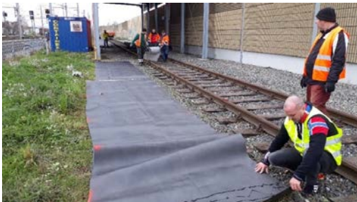
Figure 52: ÖBB-Infra Installation root barriers Nov 2018 University of Applied Sciences Carinthia
