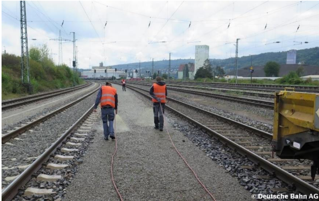
Figure 13: Biomineralisation - Preparation of working path
