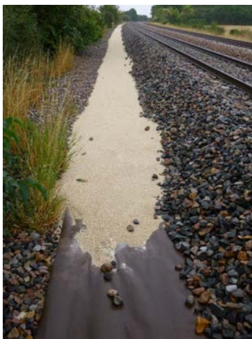
Figure 50: Geotextile laying and covering
